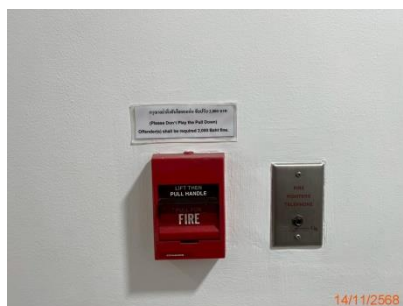
Fire Alarm Manual Station
